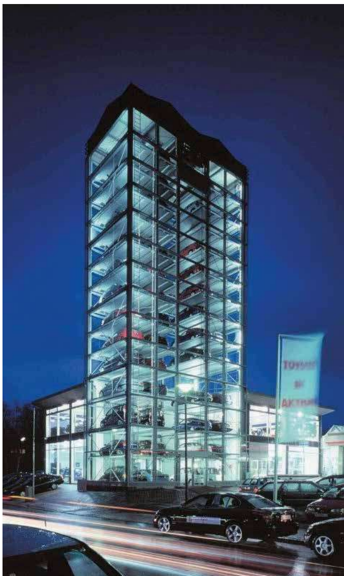
● Tower shows cars placed into parking slots
